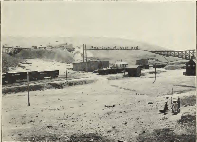
B. NELSON COAL MINE AND PLANT AT SAND COULEE, MONT.
